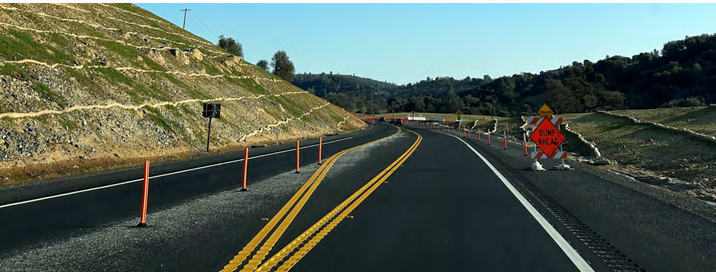
Figure 6.2 Photo of State Route 4 Wagon Trail Project
